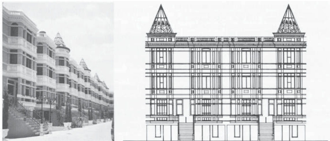
Figure 3 Chicha Castle, Bangkok, designed by architects Jira Thanaruch and Naronrit Paneenij in 1988 Note.
